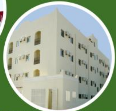
DR. HAMAD AL SULAITY G+3 STAFF ACCM. PROJECT, ST NO.2, INDUS AREA
